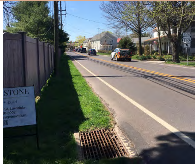
Tight spaces and utilities along PA 113 southbound
