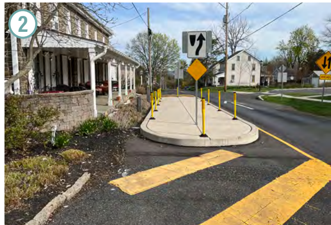
2 Traffic barrier installed on Old Skippack Road
