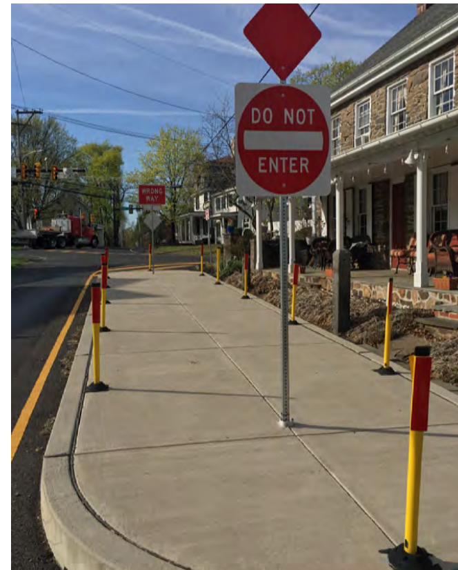
Concrete traffic island installed to block lane for one-way traffic on Old Skippack Road
