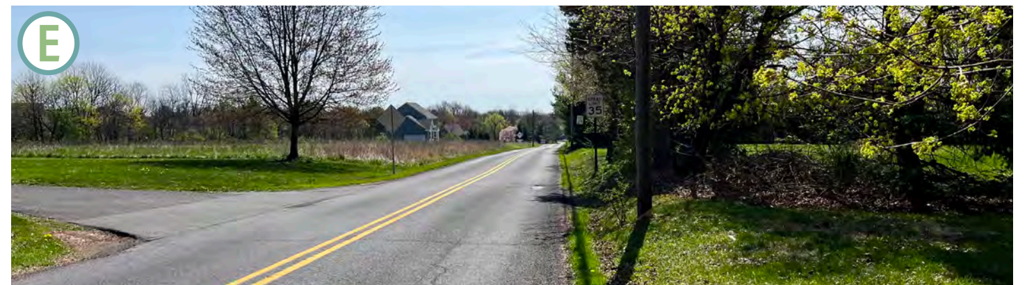
Morris Road looking eastbound away from Village Core
